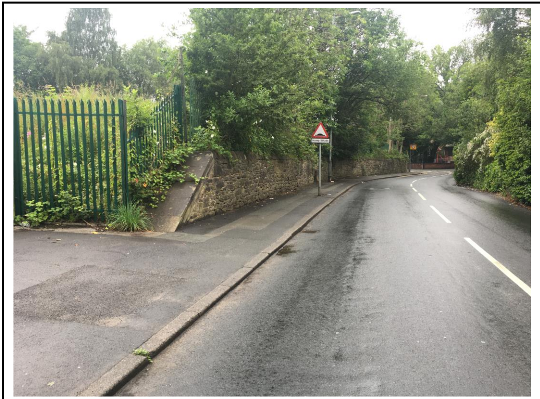
Photo 4 – Park Road (indicating stone retaining wall with planting above)
